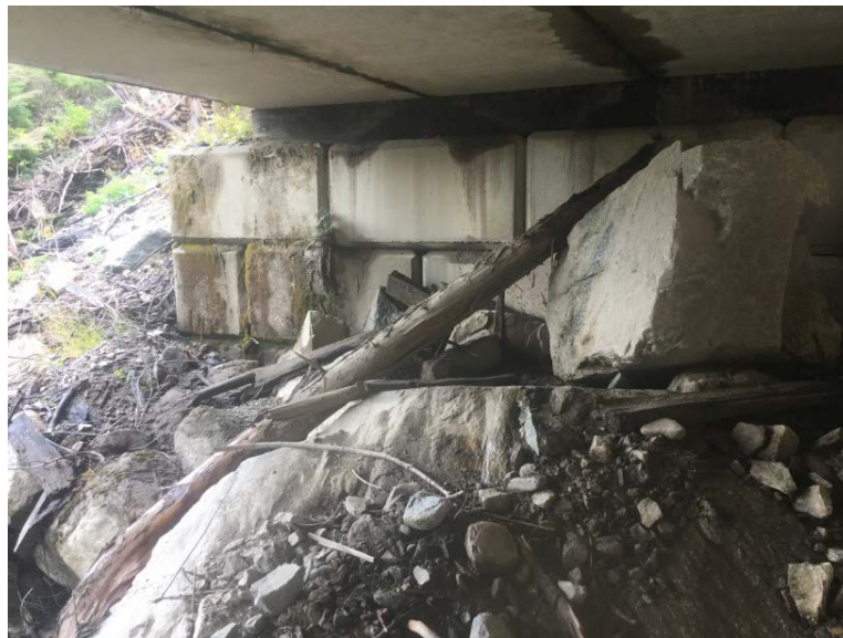
Right Bank Abutment when facing downstream
