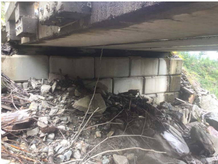
Left Bank Abutment when facing downstream
